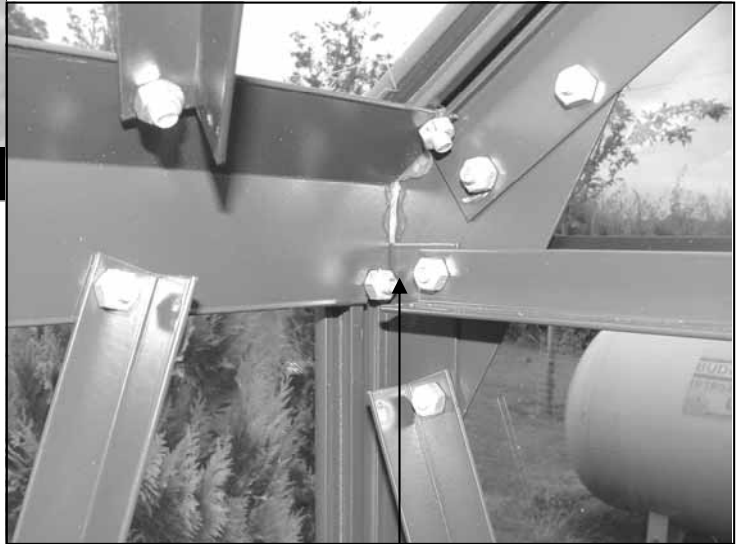
Inside eave area siliconed.
