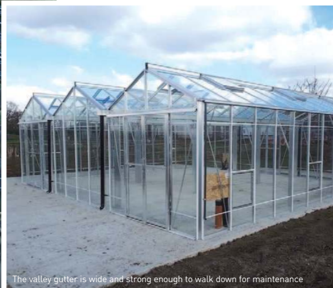
The valley gutter is wide and strong enough to walk down for maintenance
