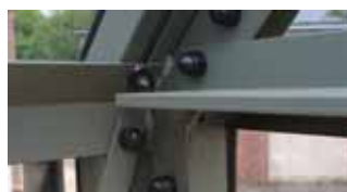
Strong Frame with box section glazing bars
